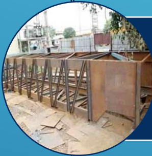
Iron Fabrication works
